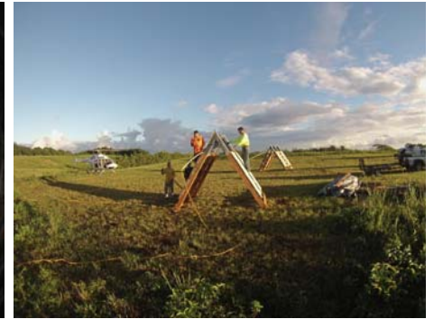
Replacement tube installed in Flume #1 and rock shields awaiting chopper lift into Honokane
