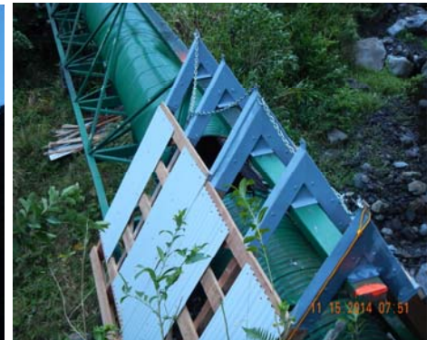
Lift into Honokane Nui by Cal Dorn and installation of new rock shields for Flume #1
