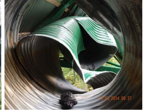
Crumpled 4' pipeline after rockfall
