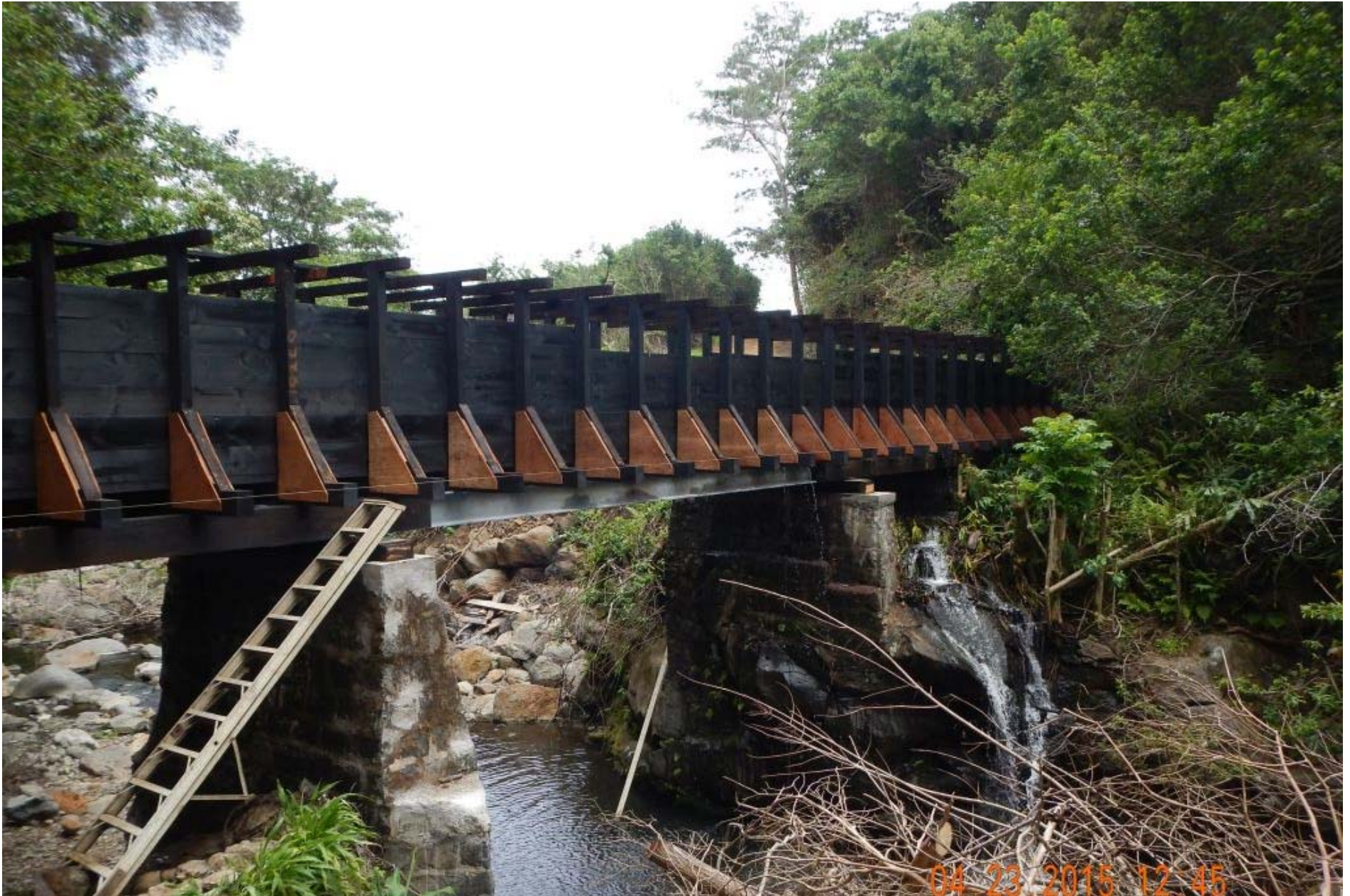
Rebuilt Flume #10 with center steel beam — April, 2015
