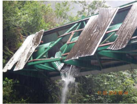
Shattered Honokane Flume #1 and rock shield
